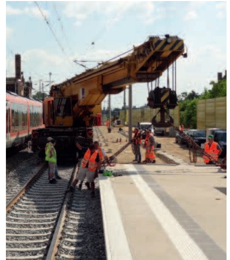
↑ Lifting concrete elements with the Multi Tasker
