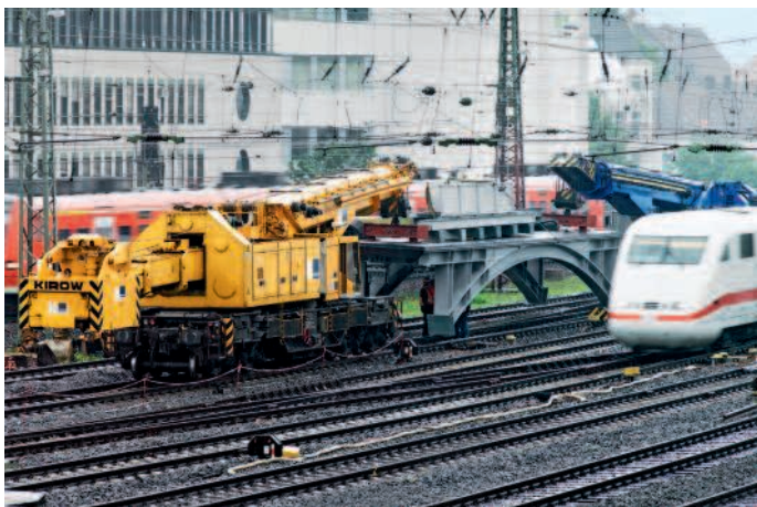
↑ Bridge construction in tandem operation
