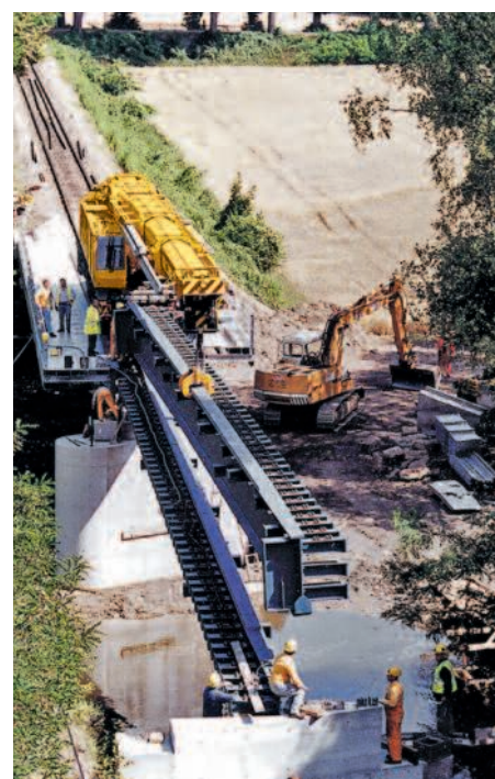
Efficient erection of bridge girders
