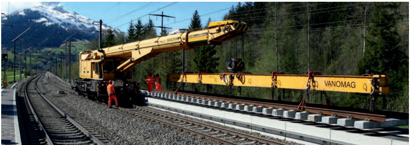
↑ Switch section lifted from the side
