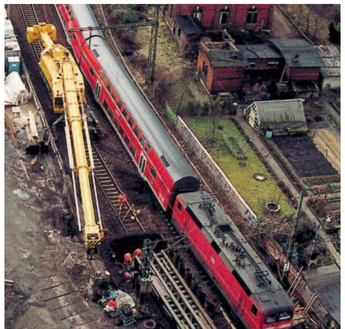
↑ The special counterweight arrangement of the Multi Tasker permits profile-free working with only one support
